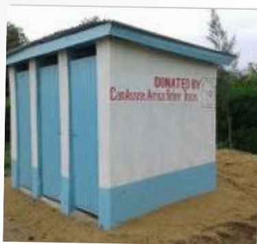
CANASSIST-FUNDED LATRINES AT THE WAMBUSA PRIMARY SCHOOL, KENYA.
