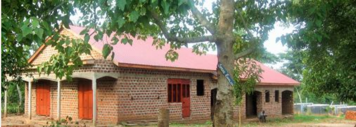
(ABOVE) NEW CANASSIST-FUNDED TEACHERS' ACCOMMODATION AND HEALTH ROOM AT HOPE FOR YOUTH SCHOOL NEAR MUKONO UGANDA.
