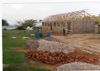
CONSTRUCTION OF CANASSIST-FUNDED SCHOOL CLASSROOMS AT A RURAL UGANDAN COMMUNITY.
