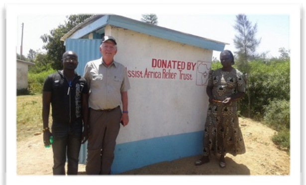
New latrine at the Wambosa School
