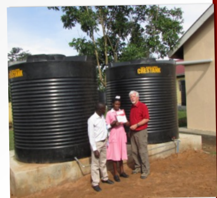
TWO OF FOUR RAINWATER TANKS INSTALLED AT OLIMAI CLINIC, UGANDA
