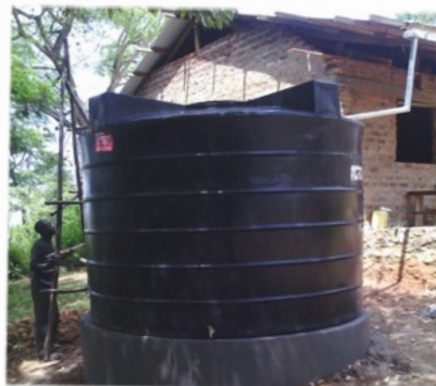
INSTALLING A NEW WATER TANK AT KAMSER SCHOOL (KENYA)
