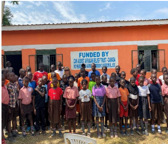
Visiting the new two classroom block at the Great Challenge School in Kampala.
